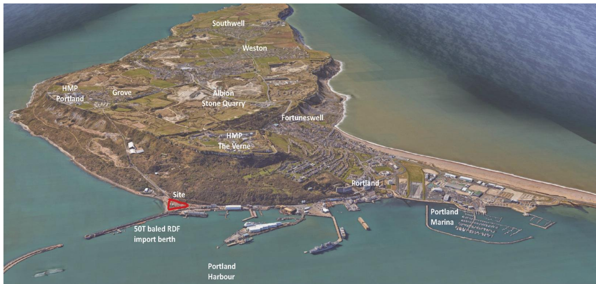
Figure 1.1 Site Location, Shown by the Red Boundary, Portland
